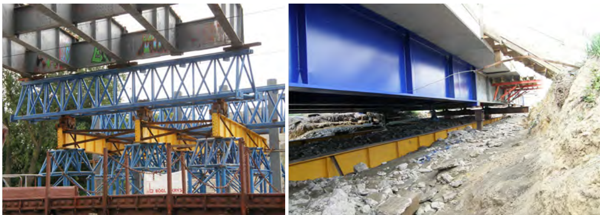
Fig. 6. Falsework as a temporary framework with launching gantry
