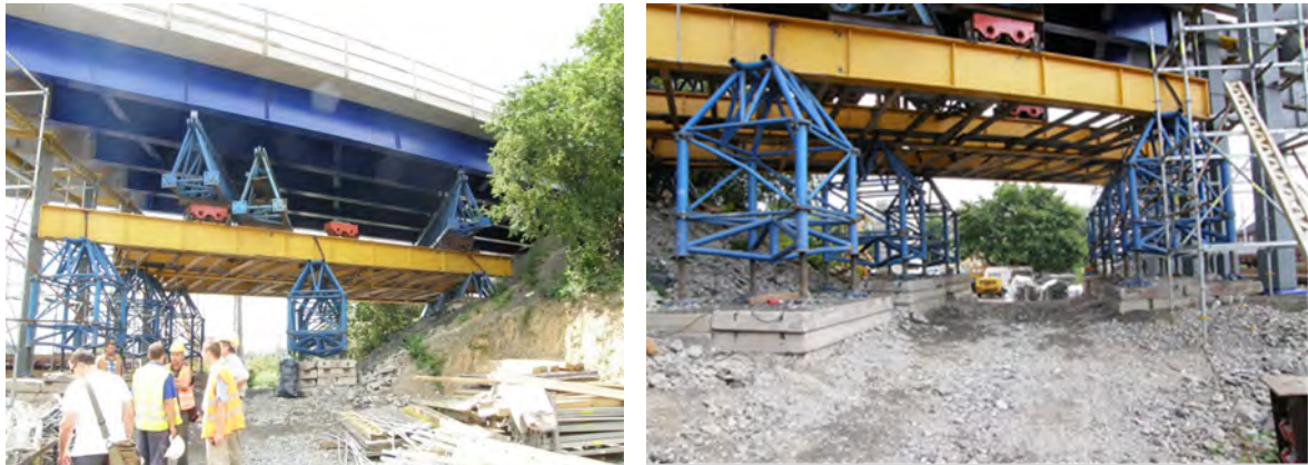
Fig. 7. Launching procedures and critical posts laying only on concrete plates
