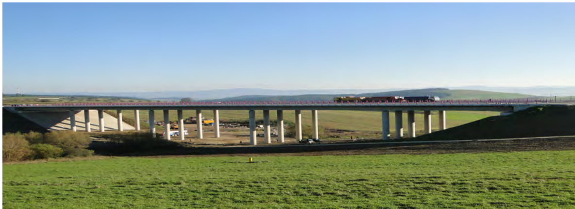
Fig. 1. Bridge structure during loading test of collapsed span
